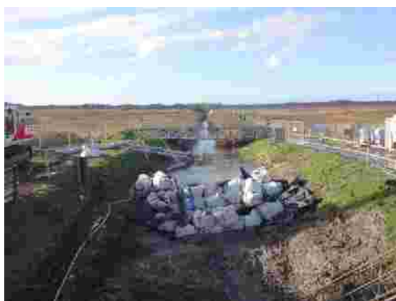
View up the New Cut with ballast bag dam
