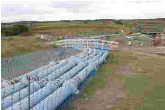
5 discharge tubes from sluice site
