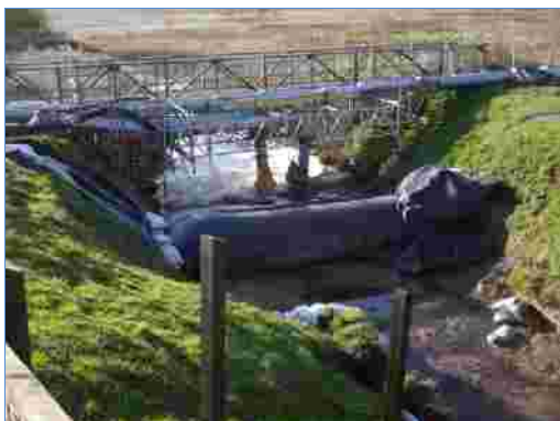
Leiston drain with Aqua dam
